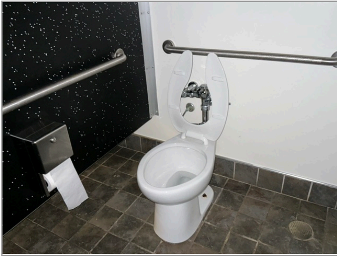
TOILET STALL OVERVIEW
